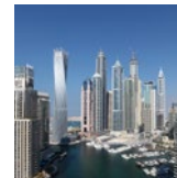
DUBAI Saving energy in air conditioning systems
